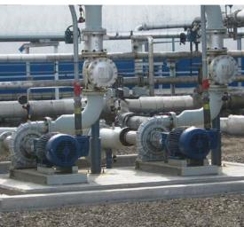
Roto-Prime® self-priming centrifugal pumps are specifically designed for pumping petroleum products, petrochemicals and solvents. The Roto-Prime design incorporates a variable capacity vane pump which quickly and automatically evacuates air and vapor, making the pump ideal for loading and off-loading transports and stripping hoses.
